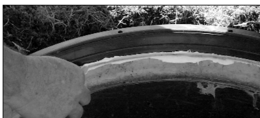
Applying adhesive fillet to inside of riser
