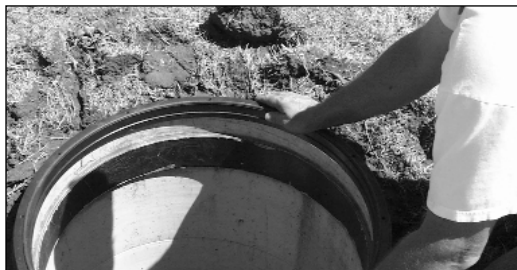
Placing RLA adapter onto riser
