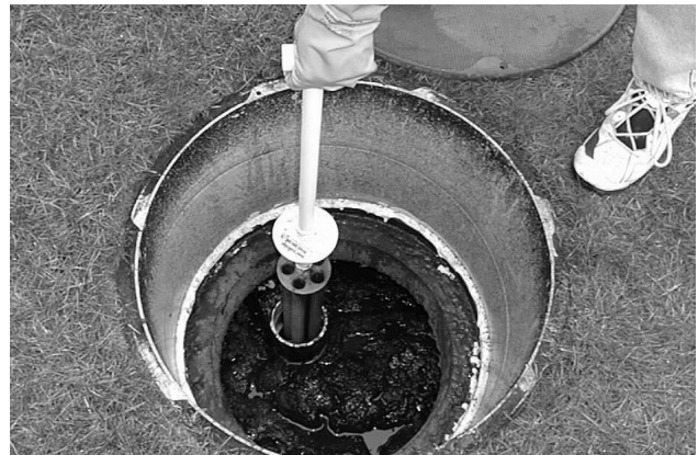
Photo 1. Remove the filter cartridge by lifting it out of its housing.
