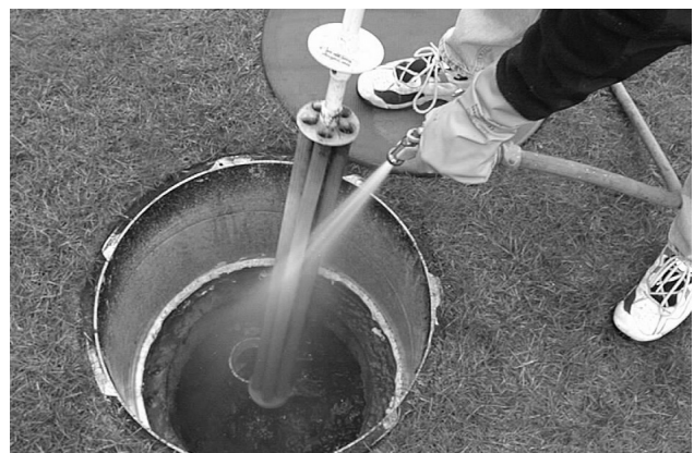
Photo 2. Spray the cartridge tubes with a hose.
