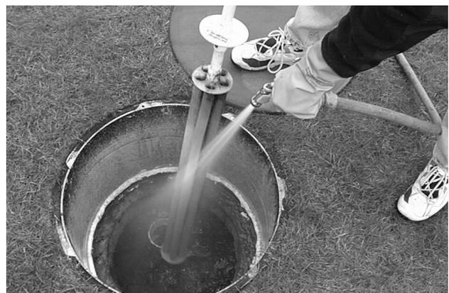
*Photo 2. Spray the cartridge tubes with a hose.*
